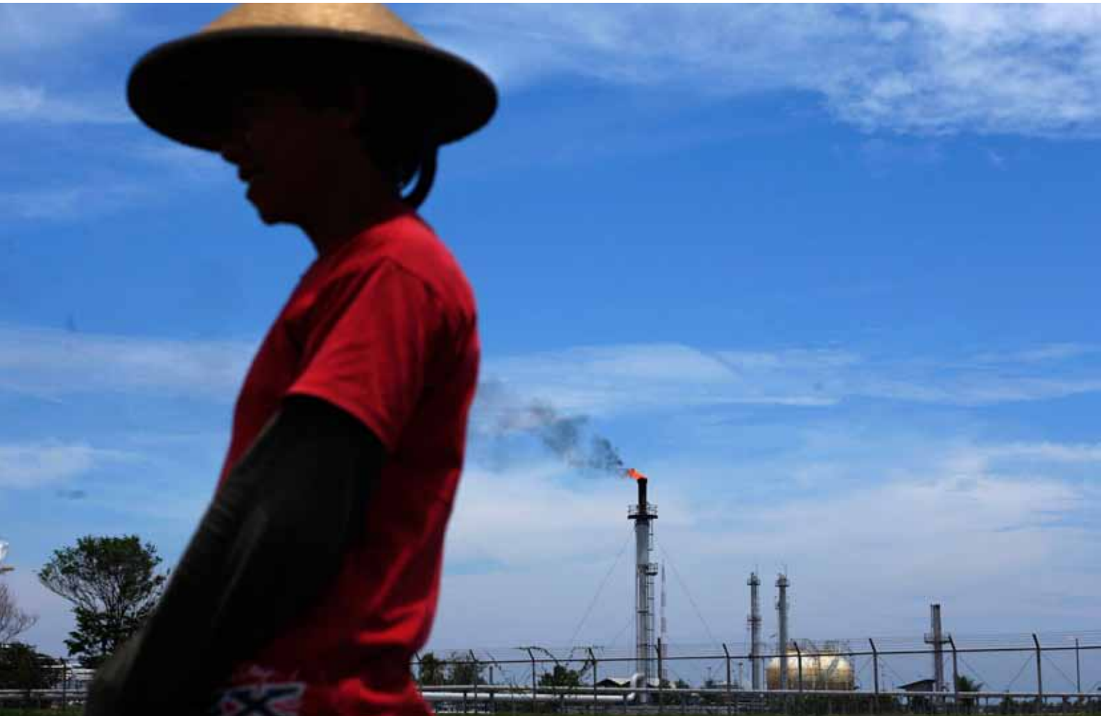
A villager works near the gas pipelines of the Cimalaya Onshore Receiving Facility owned by Indonesia state oil and gas company Pertamina near Subang, Indonesia's West Java Province. REUTERS/Beawiharta
