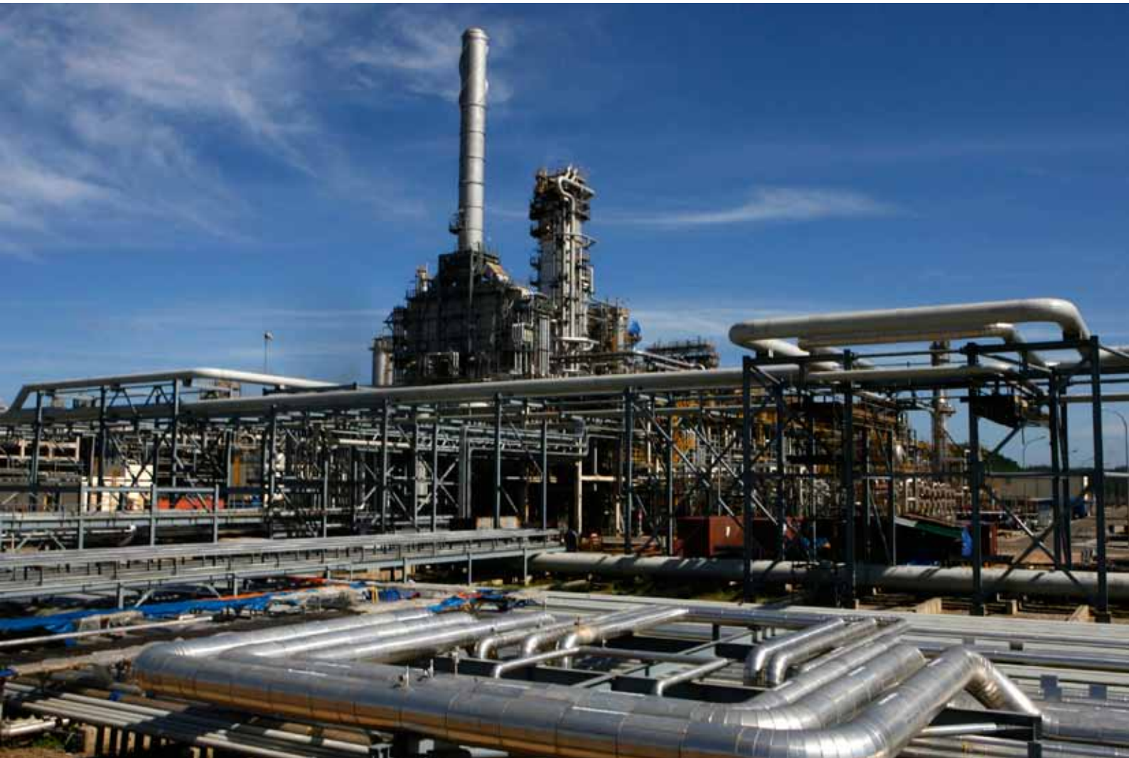
A general view of Dung Quat oil refinery plant in Vietnam's central Quang Ngai province. REUTERS/Kham
